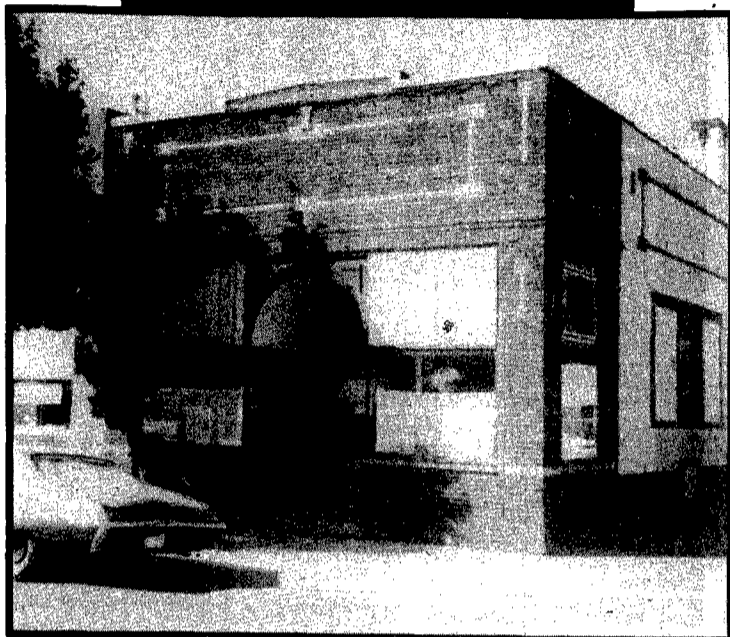
THE JOB SITE, 110 Main Street
